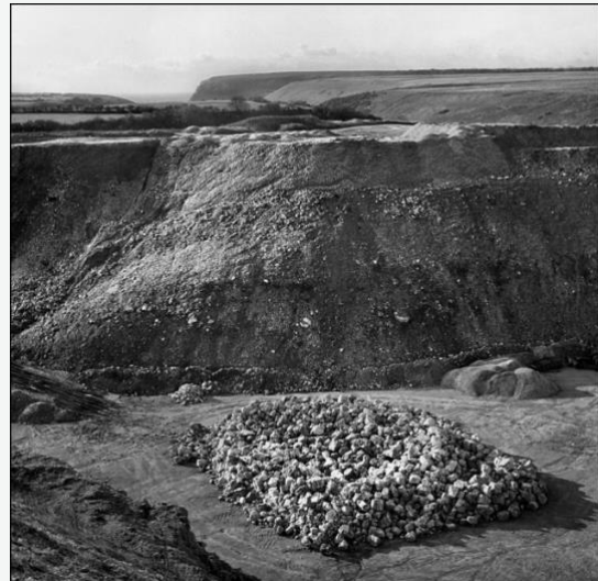
Gabion/cage stone and Rock Armour/ Sea Defences
